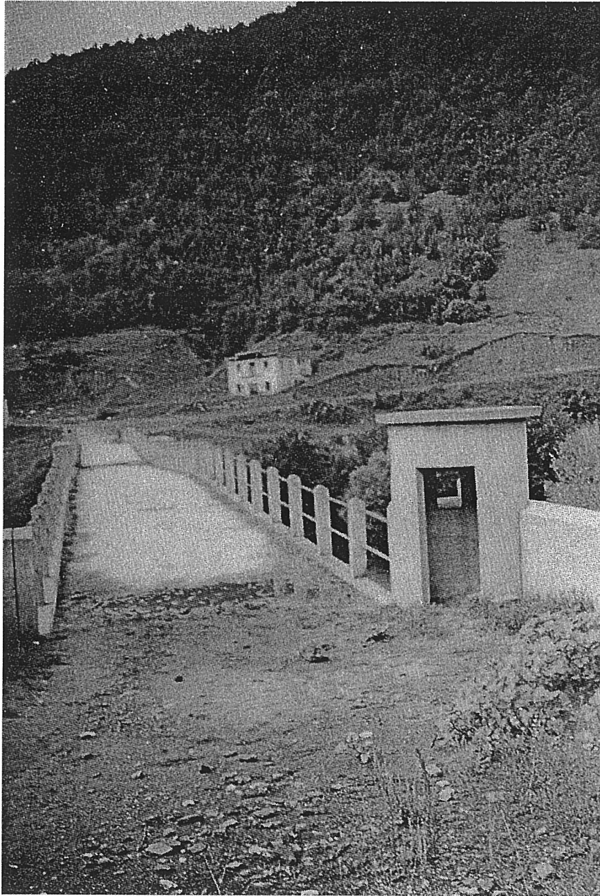
Bridge over the Nestos.
